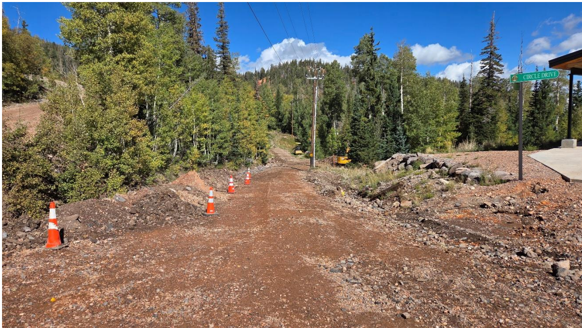
Connection between Circle and Gurr Well looking down toward Bobcat from Circle
